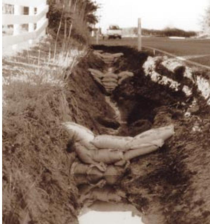
**Sandbags used to control drain velocity.**
