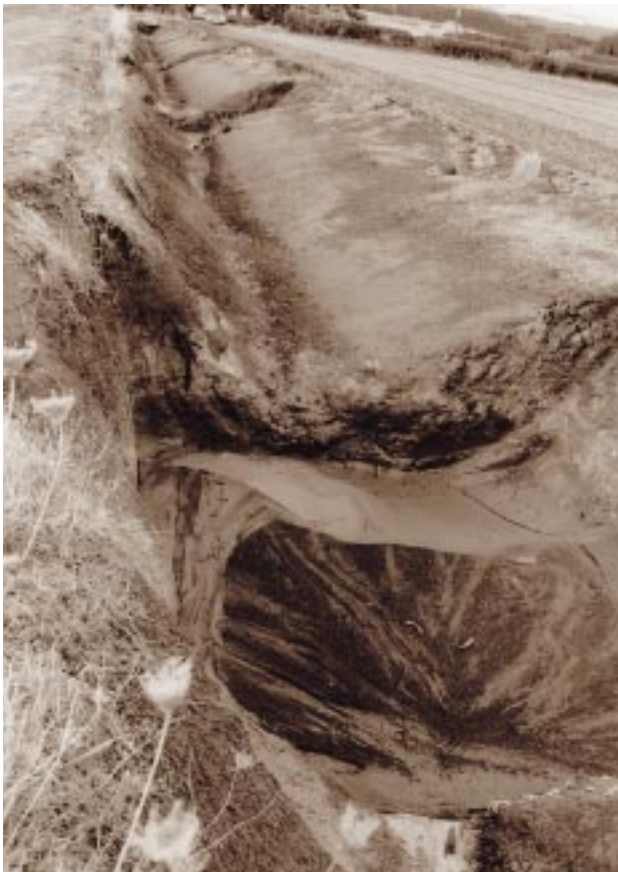
Silt traps. Photo: Franklin Sustainability Project.
