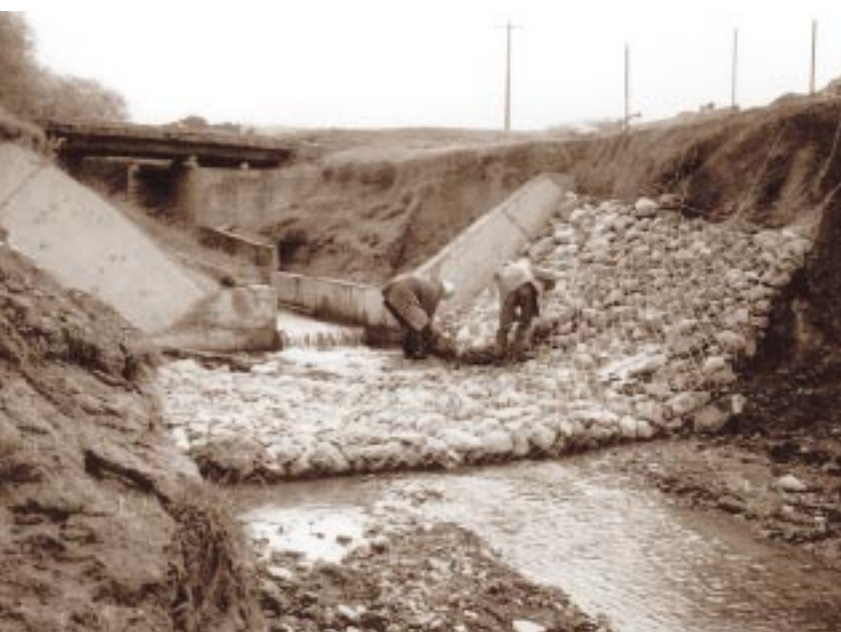
Rock gabion drop structure.
