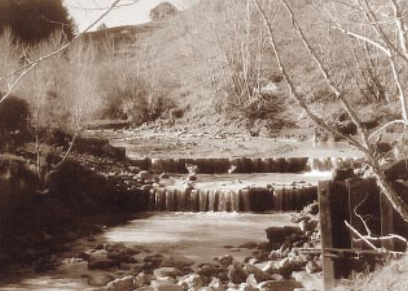
Sheet piling drop structures.
