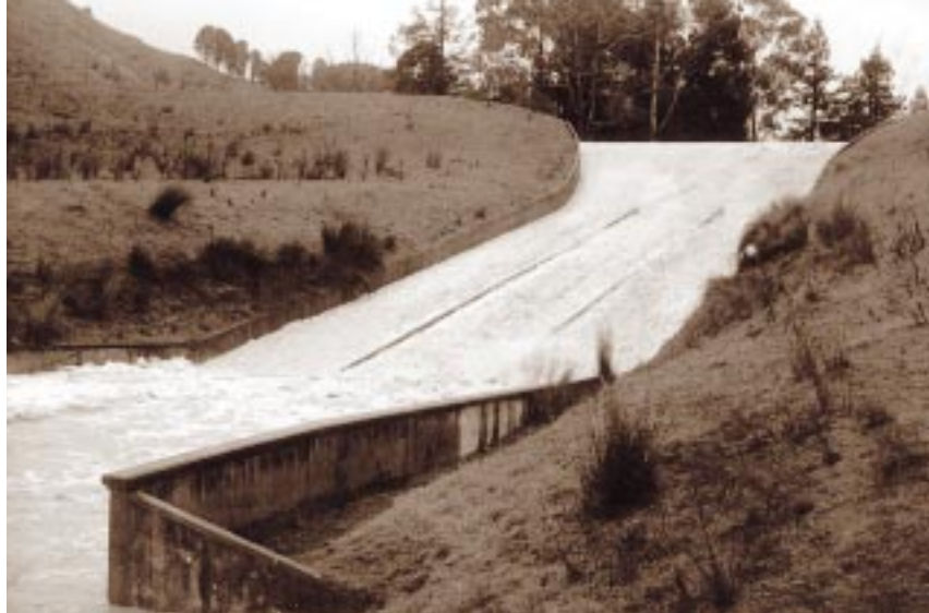
Concrete drop structure – spillway over dam.
