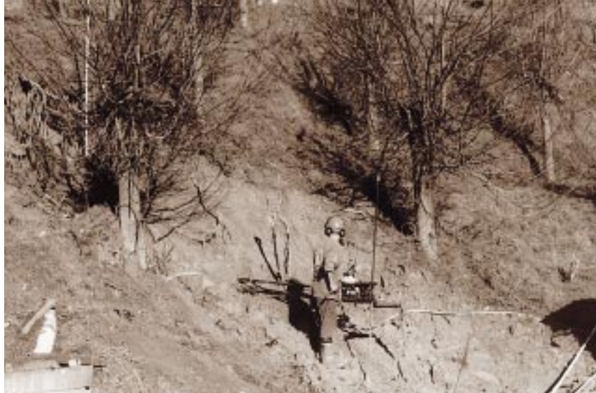
Portable drilling equipment used to install horizontal bore draws. This bore produced an initial flow of approx 3,500L per hour and prevented further slope instability.
