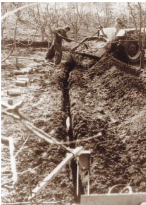
Installation of tile drains through orchard.
